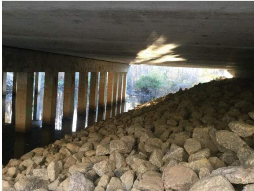
Underneath SC 707/Collins Creek Bridge – looking downstream
