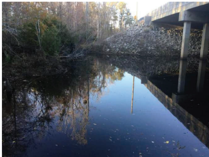
Downstream Face of SC 707/Collins Creek Bridge – looking at right overbank
